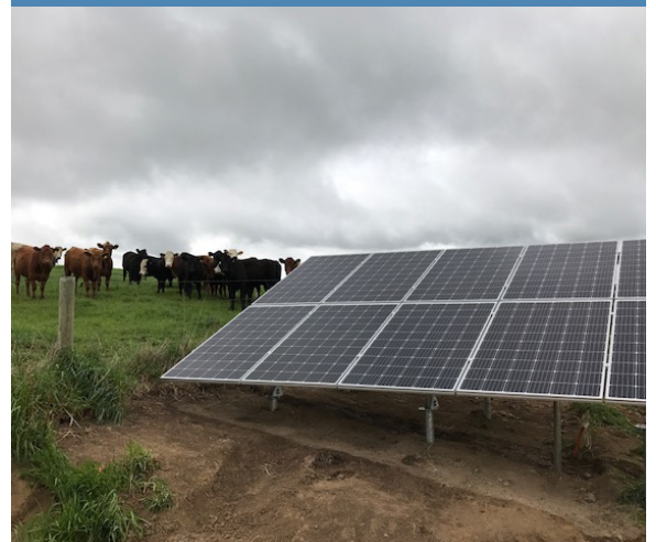
PHOTO: Fish Creek Off Grid System VIC. 15KW.
